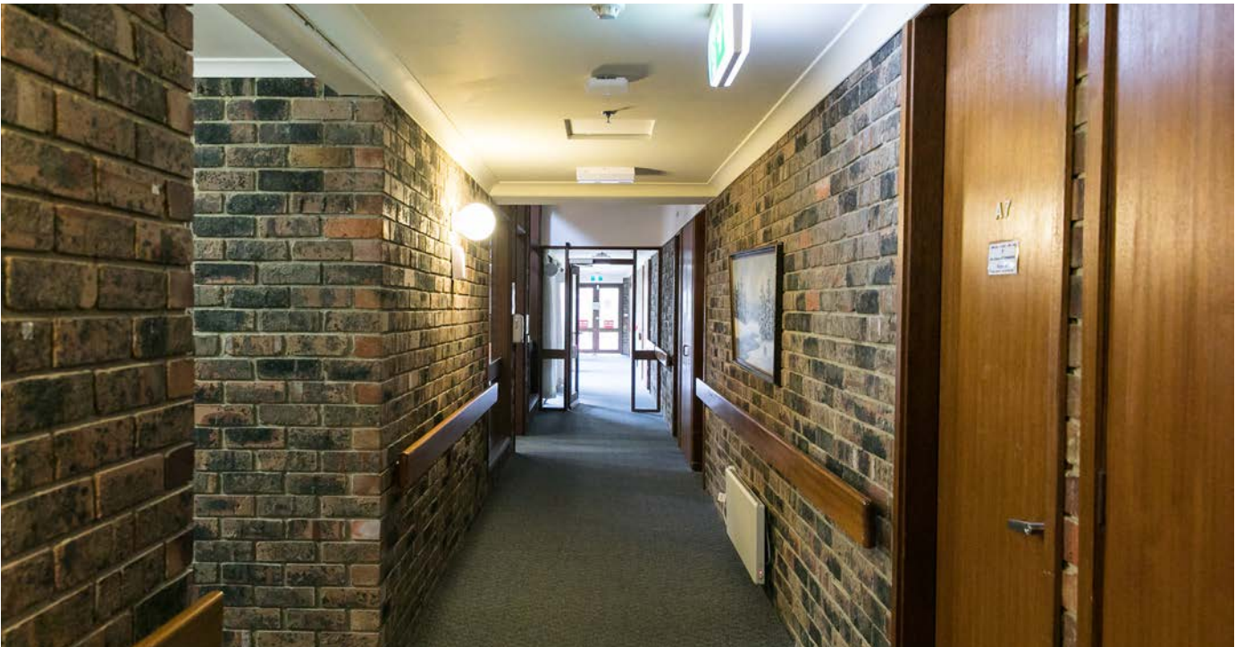
Circulation areas in the serviced apartments are generally non compliant with current accessibility standards.
