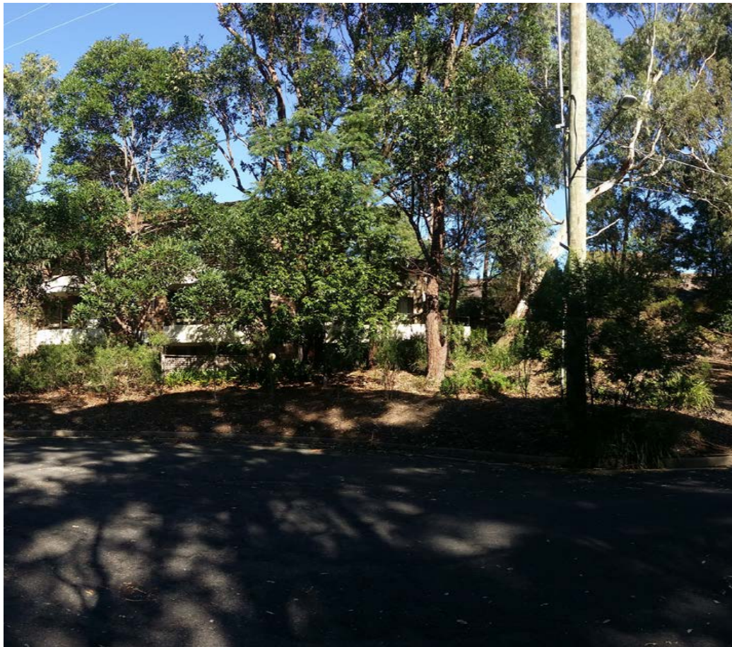
View of embankment along Stanhope Avenue
