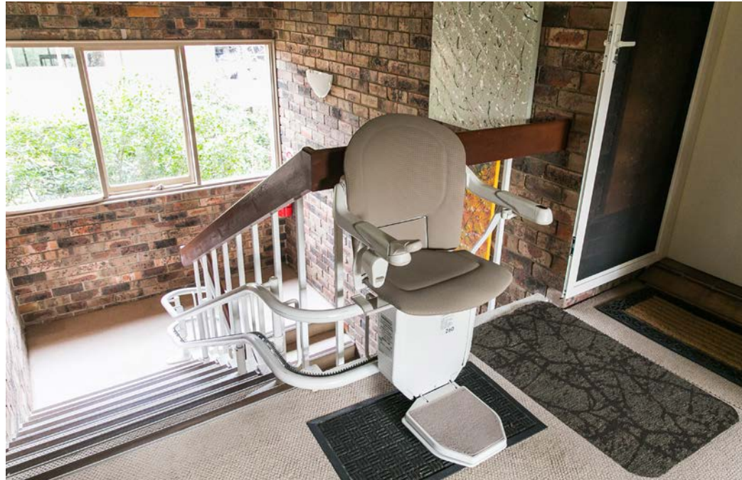
In the absence of lifts in buildings, stair lifts are used to move residents between levels.
